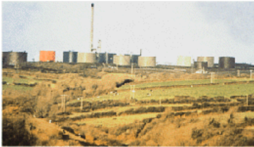
12 A large oil tank farm at Milford Haven, Pembrokeshire, Wales. The tanks have been painted a range of receding colours, some to create shadow effects. The one red tank acts as a focal point (an accent colour) which draws the eye and helps pull the composition together. (Courtesy of Ray Perry.)
